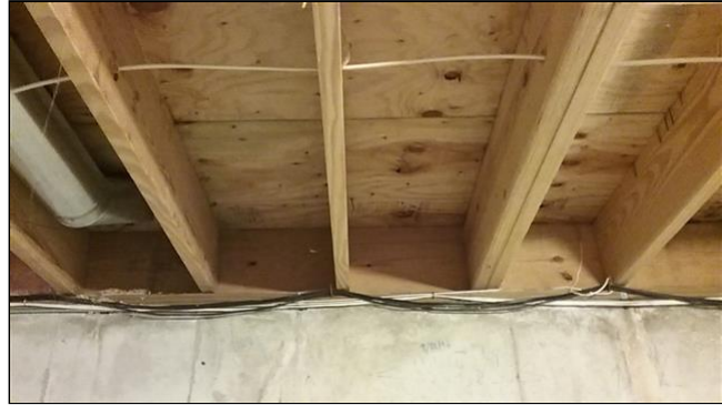
Wood Floor Joists
