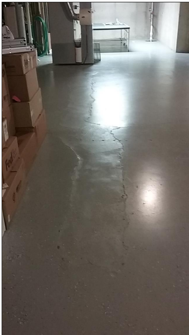
7.2 Item 1(Picture) Prior Floor Drainage Repair
